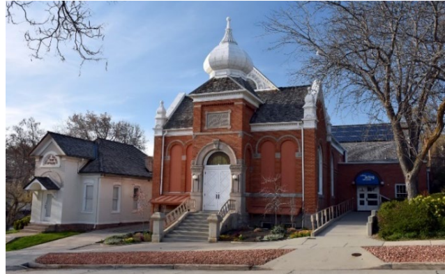
Photo above: After decades as a house of worship, the building at 168 W. 500 North has been home to Salt Lake Acting Company since 1982, housing two theaters, rehearsal space, dressing rooms, a box office and more.
